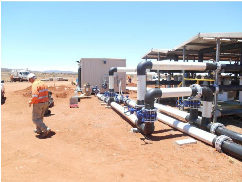
Figure 2: Installation of FME Wellhouse 1 and filter skids
