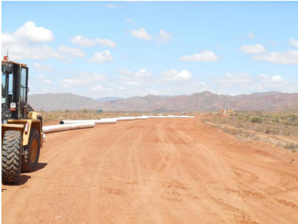
Figure 3: Preliminary laying of FME trunkline, prior to welding
